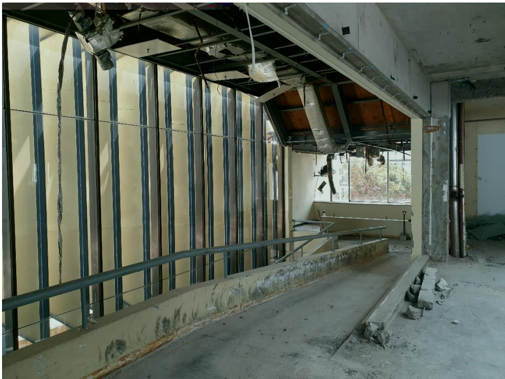
Photo 18: View of Light Well & Ramp (looking North) on Level 2 of Administration Building.
