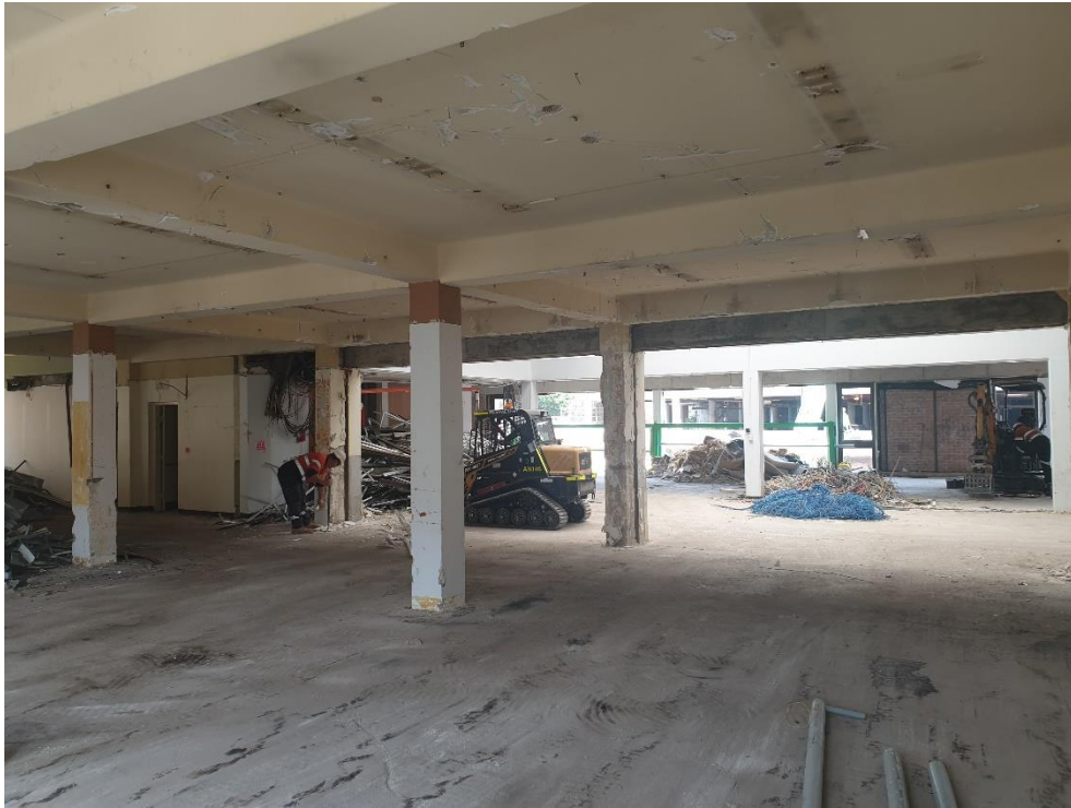
Photo 17: View looking South on Level 2 of Administration Building. Note soft strip demolition complete on this level and waste materials segregated and stockpiled.
