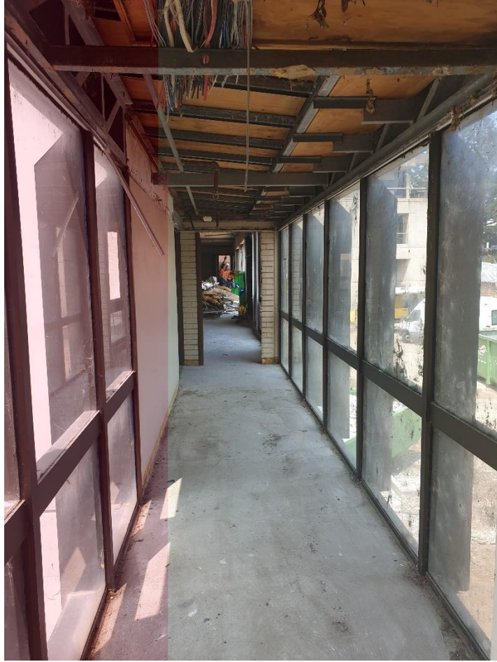
Photo 15: View within Level 2 Connection Corridor of Administration Building looking East. Note soft strip demolition completed.
