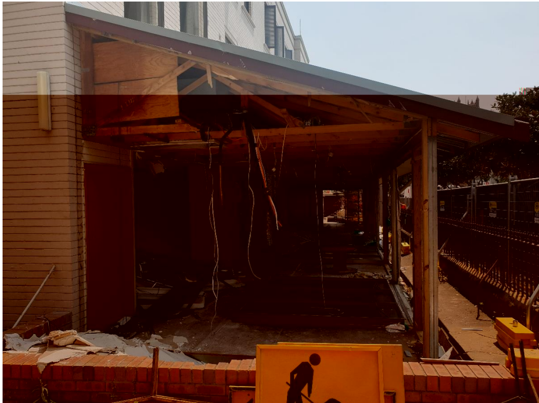
Photo 04: View (facing West) of lightweight structure attached to Administration Building. Demolition works underway to allow erection of scaffold.
