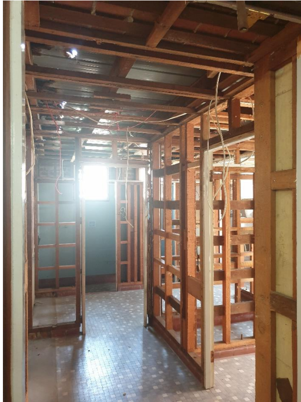
Photo 13: View of existing Jury WC/Showers in Heritage Building. Asbestos removal works completed within Existing toilets
