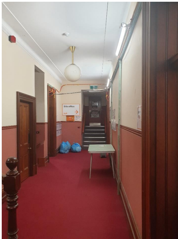
Photo 14: View of connection doorway to Administration Building from G07 in Heritage Building. Note temporary lighting and power installed for Site Offices.
