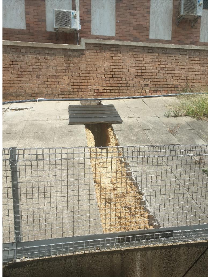
Photo 10: View of investigation works at South West Buttress being completed to for piling design
