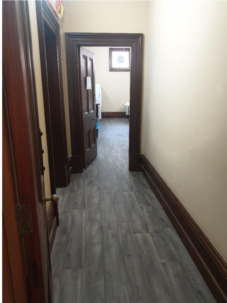
Photo 12: View of existing Jury Room 3 in Heritage Building. Floor coverings removed and replaced with vinyl to be used as Site Lunch Room.
