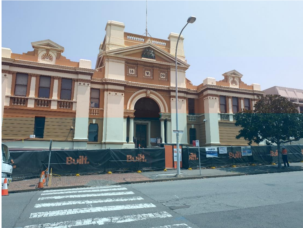
Photo 02: View of site from Corner of Bolton and Church Streets facing South.
