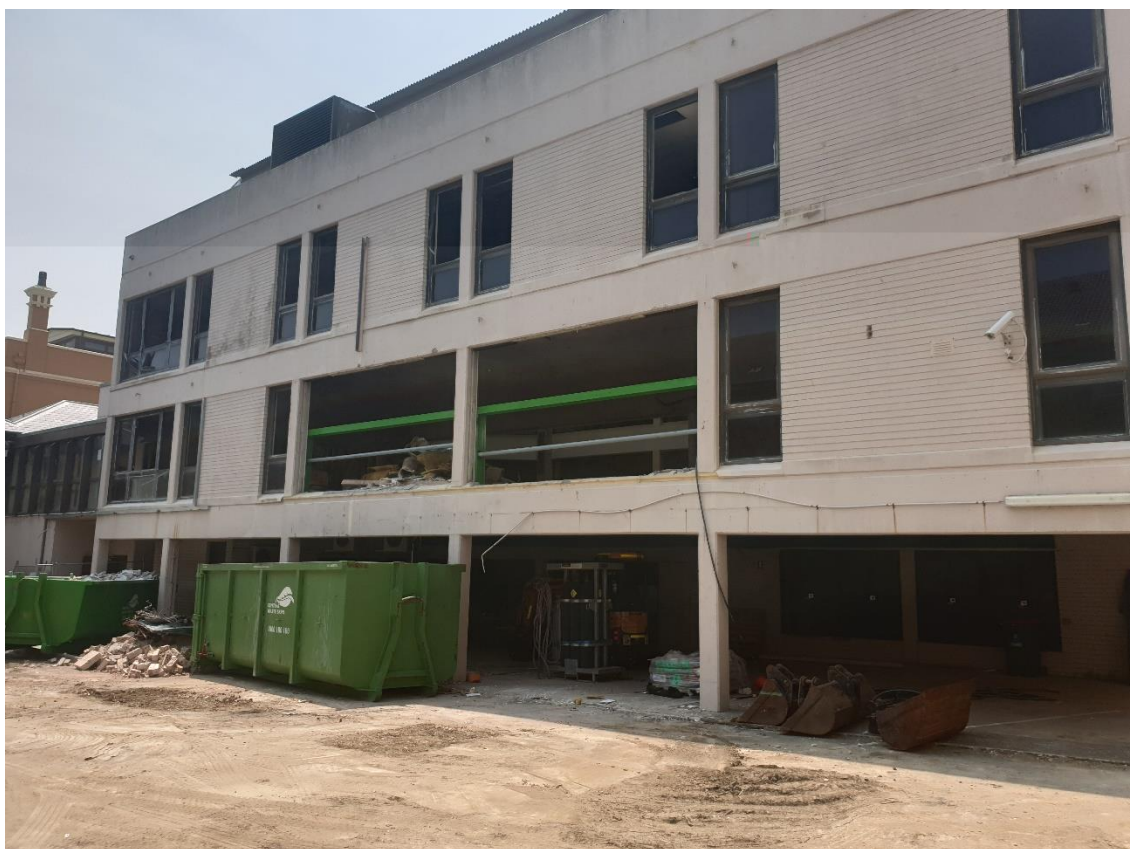
Photo 05: View of Southern façade of Administration Building from rear of site.
