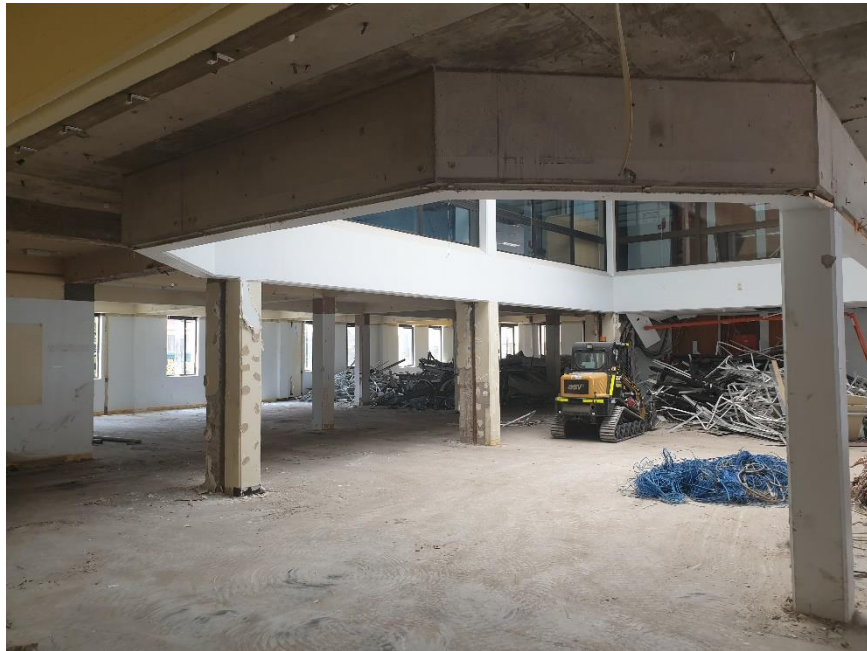
Photo 16: View looking North East on Level 2 of Administration Building. Note soft strip demolition complete on this level and waste materials segregated and stockpiled.
